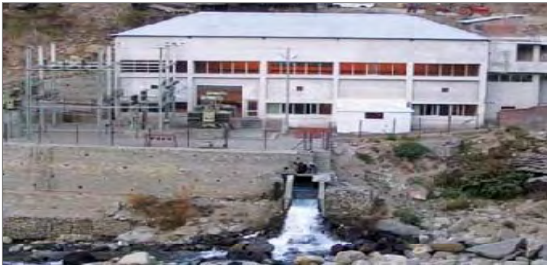
Figure 10: Aleo Small Hydro (3MW) Power Project in Himachal Pradesh Source: MNRE website
