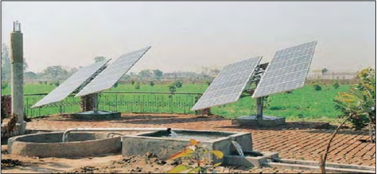
Figure 13: SPV water pumping system in Punjab
